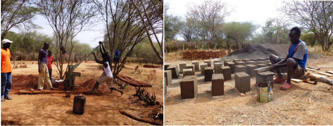
Making bricks and blocks for our new visitor huts.
